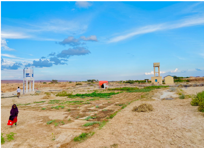
Rehabilitation and solar installation of Mindhicir borehole in Sanag region
