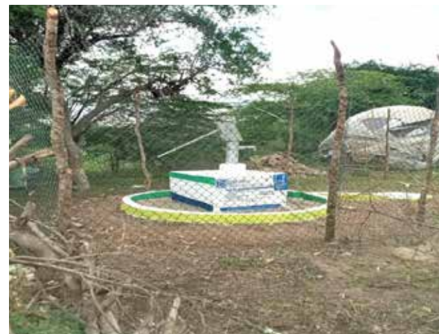
Rehabilitation of shallow wells in the outskirts of Jowhar town, Hirshabelle Sate, Somalia
