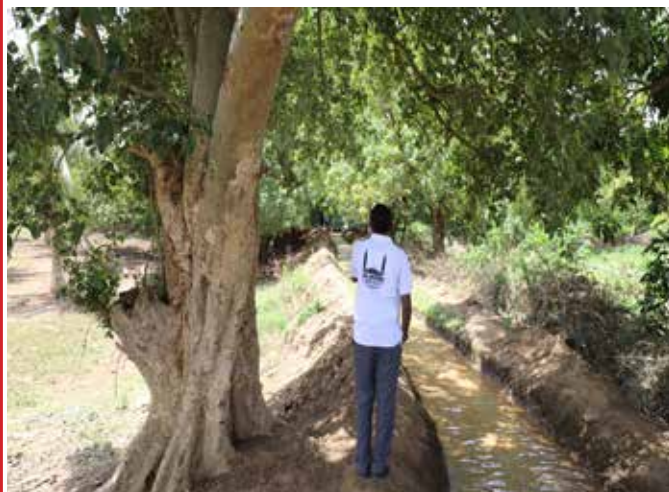
Rehabilitation of 2 irrigation canals in Mareray, Afgoye- Somalia
