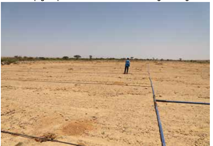
Installation of drip irrigation system for 12 farms in Puntland
