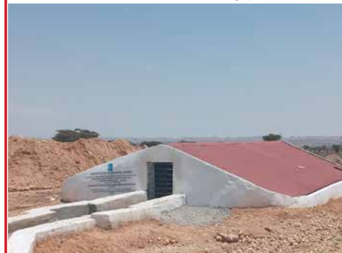
Construction of communal berkads in Bixin village
