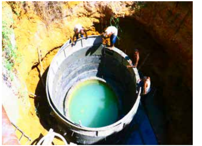
Rehabilitation of a shallow well in Jalelo village, Somaliland
