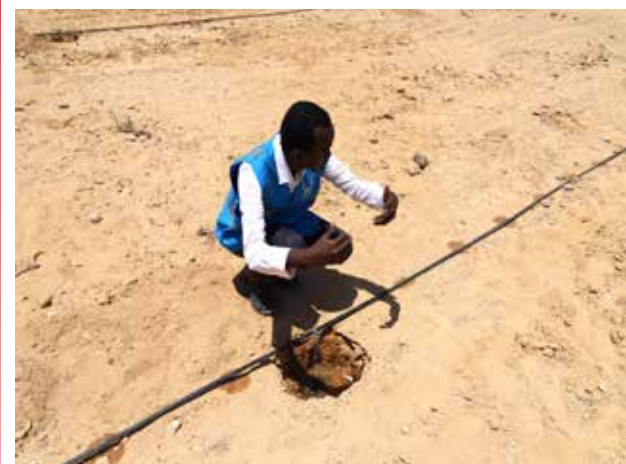
Installation of drip irrigation system for 12 farms in Puntland
