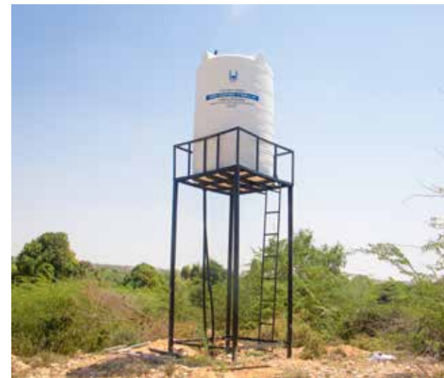
Construction of a water tank in Jaleelo village, Somaliland
