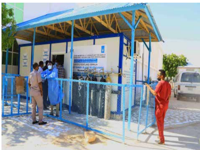
IRS installs Oxygen Plant in Qardho General Hospital-Puntland
