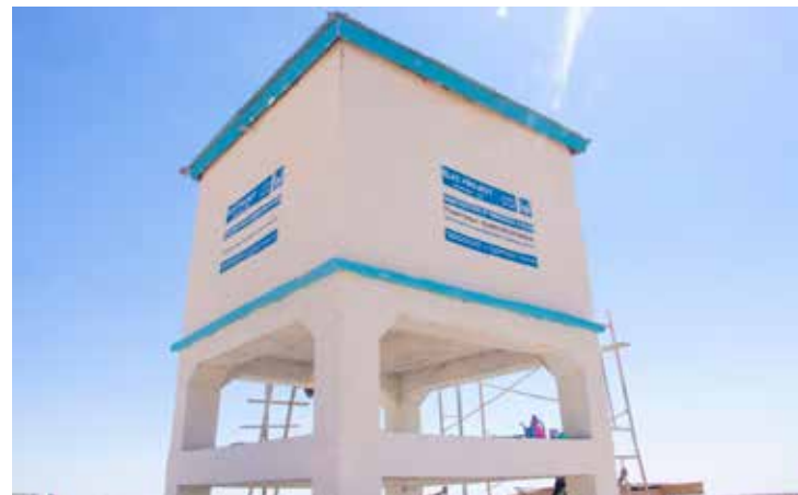
Islamic Relief Constructs mini water system in Kalmac village, Somaliland
