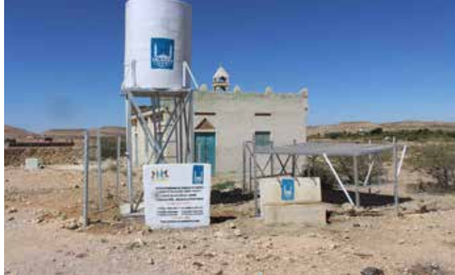
Islamic Relief completes the construction of water facility in Rabable village, Puntland
