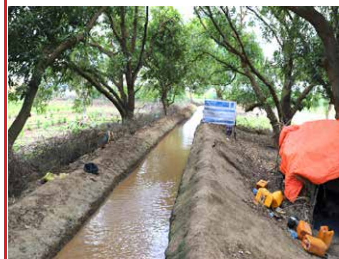
Rehabilitation of 8km canals in Afgoye, Somalia
