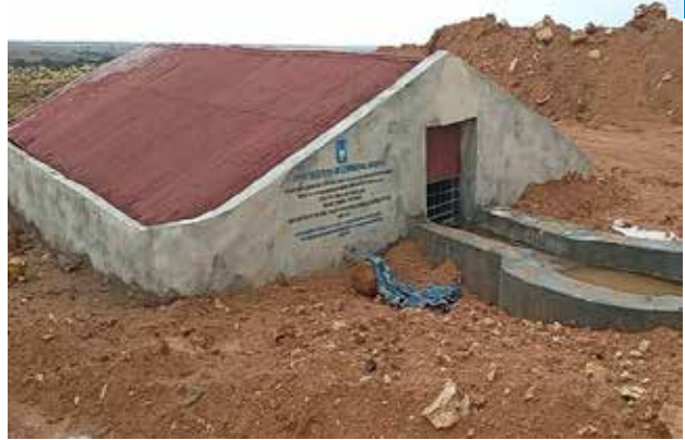
IRS completes the construction Berkads in Ceel Laman village of Somaliland
