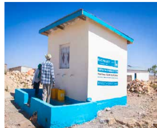
Construction of mini water system in Kalmac village, Somaliland
