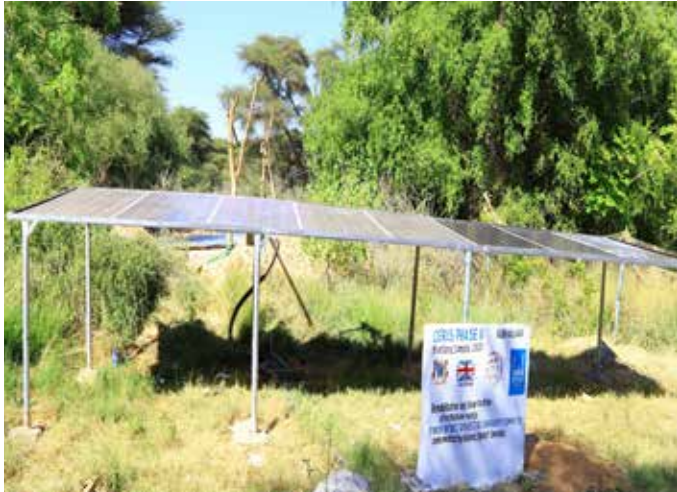
Rehabilitation & solarization of four shallow wells in Kubo village
