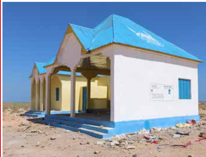
IRS constructs cooperative blocks in Kulule, Gumbah and Handa villages of Puntland, Somalia
