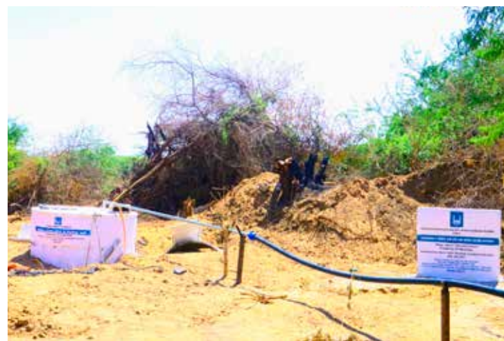
construction and rehabilitation of a shallow well in Jaleelo, Somaliland
