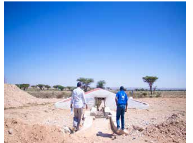
Construction of communal berkads in Bixin village
