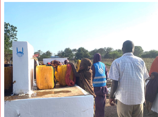
Drilling and equipping of a new borehole in Jowhar district, Middle Shabelle region, Somalia
