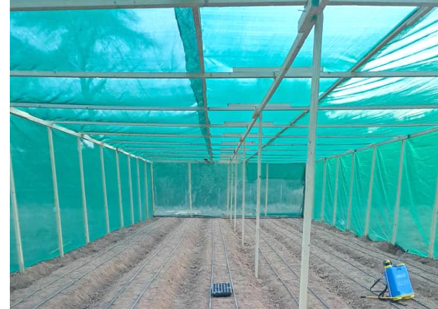
Installation of greenhouses in Kubo village of Puntland, Somalia
