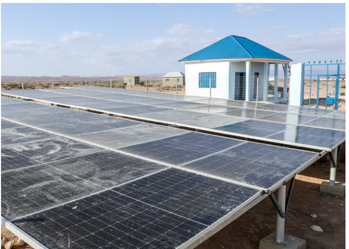
Drilling and equipping of a new borehole in Wardher village, Puntland.
