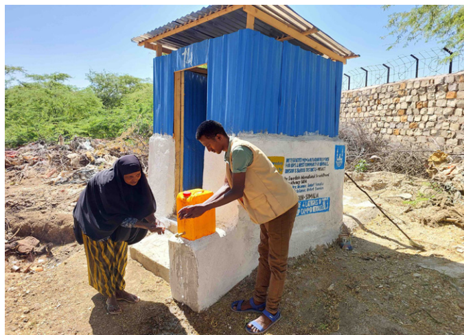
Construction of 20 latrines to the droughts affected families in Berdale
