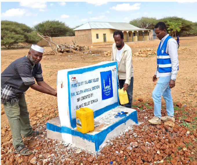
Rehabilitation of Jalam\Bandar borehole in Puntland, Somalia
