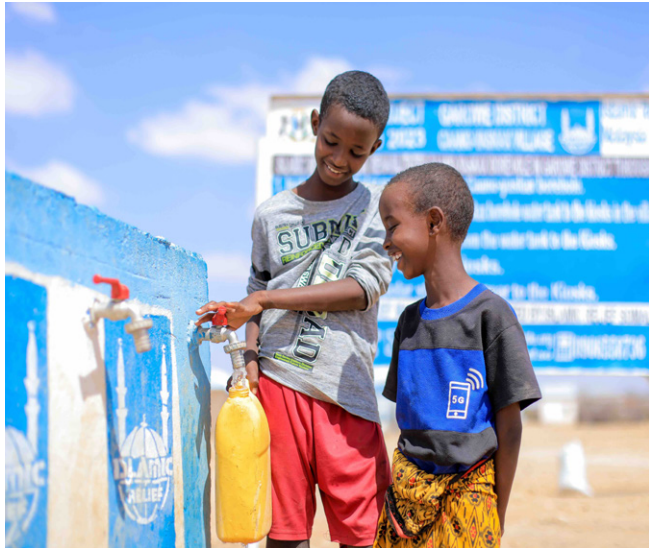
Children collecting water from a newly constructed water kiosk in Anoyask village in Puntland, Somalia
