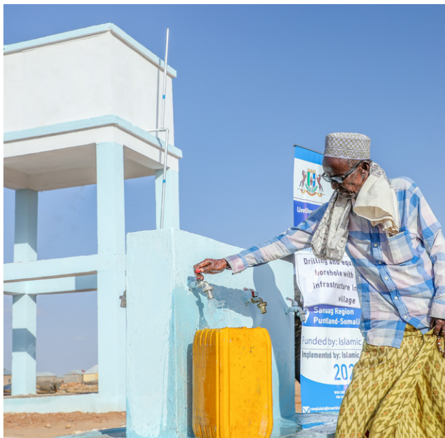
Drilling and equipping of a new borehole in Wardher village, Puntland
